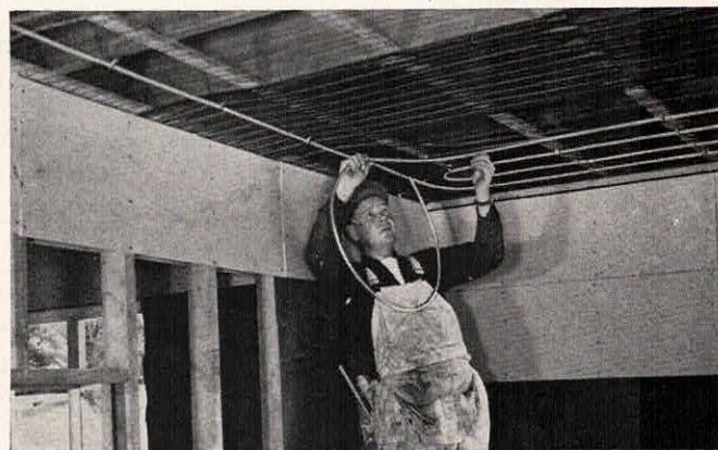
Making uniform bends by hand, to the required center-to-center distance of tubes, using a helical spring to bend the tube.
